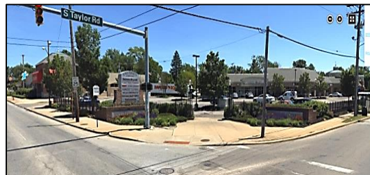
Southeast Corner of the South Taylor Road and Cedar Road Intersection
