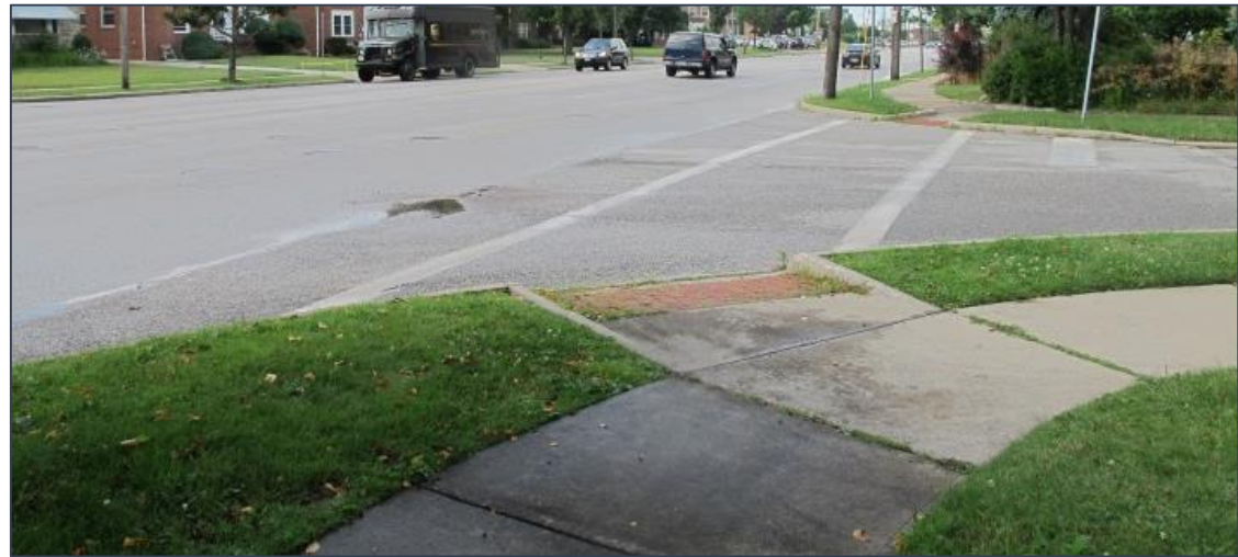
Picture 9: Typical ADA-compliant curb-cut ramp with brick-style truncated domes
