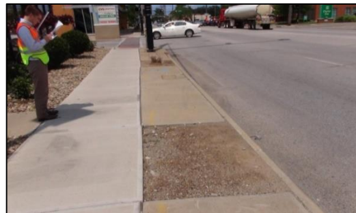
Empty buffer on the west-side sidewalk next to Boston Market on Warrensville Center Road south of Cedar Road
