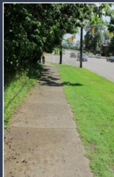
Picture 3 Warrensville Center Road east-side sidewalk north of Meadowbrook Blvd.
