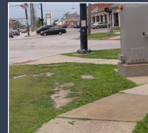
Picture 6 Warrensville Center Road at Washington Blvd. sidewalk continuity at the southeast corner
